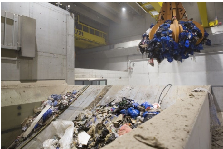
Fig. 4: On certain days, up to 700 tons of waste reach the EZF. After incineration, even the residues contain numerous raw materials that can be reused. In this way, the power plant recovers about 50 kilograms of mercury, 1.5 tons of lead, 60 tons of zinc and one ton of cadmium annually.
